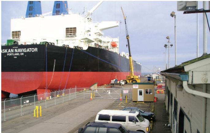
Figure 43. The Port's Terminal 1, originally built for forest products export, now primarily supports large vessel topside repair and cruise ship stop-overs.
