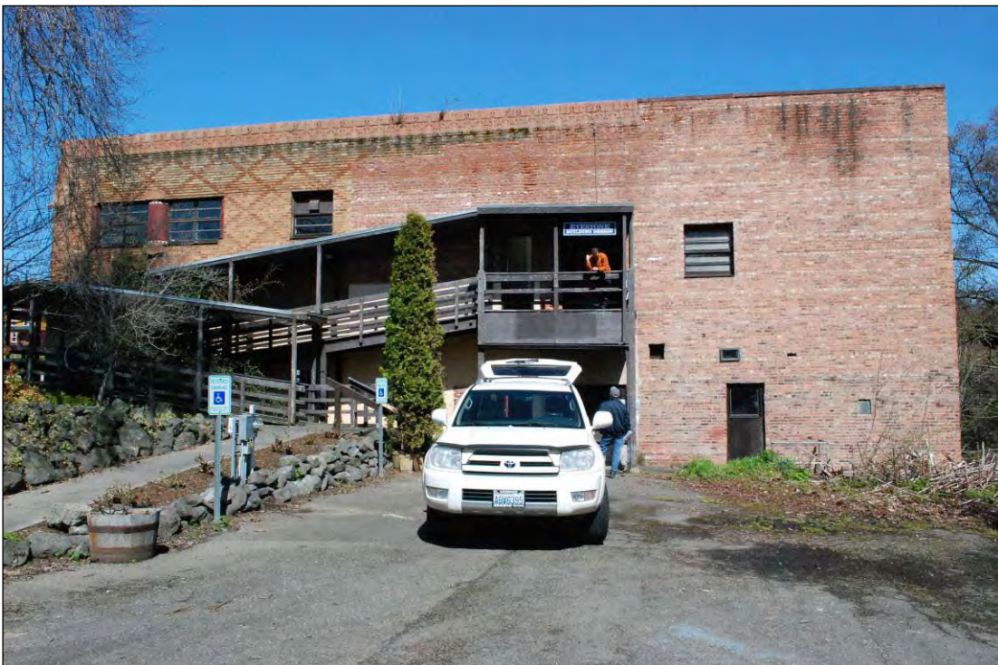
Figure 5 Below: View of building from the south (April 2011)
