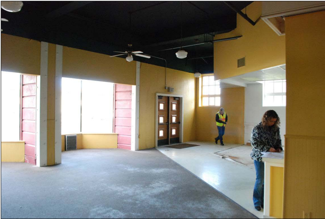
Figure 18 Above: Overall view of ground floor interior space looking west (April 2011)
