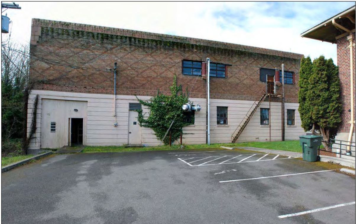
Figure 3 Below: View of building from south (April 2011)
