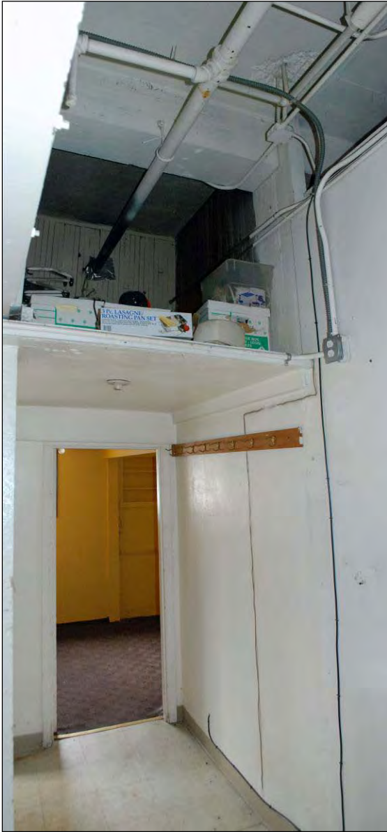
Figure 30 Left: View of ground floor corridor, looking south (April 2011)
