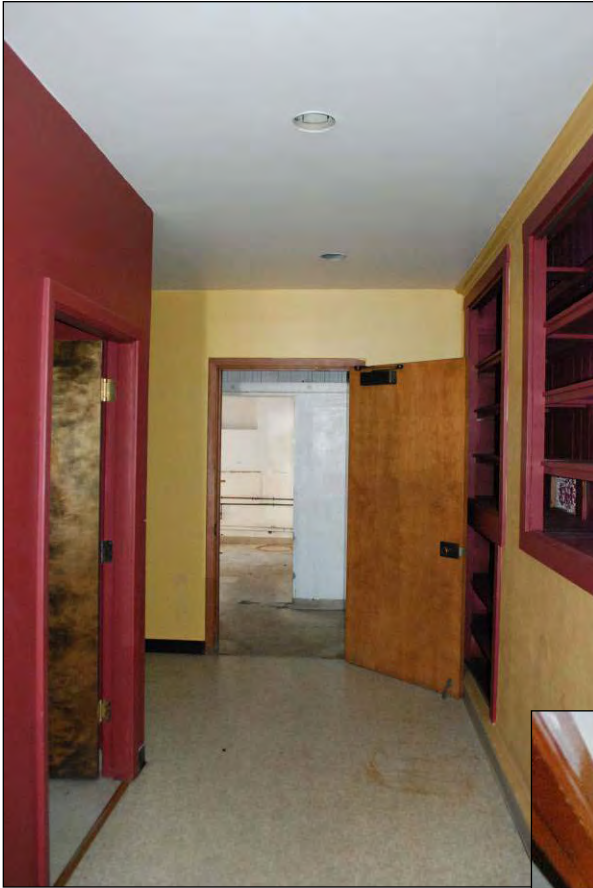
Figure 22 Left: View of ground floor hall, looking east (April 2011)
