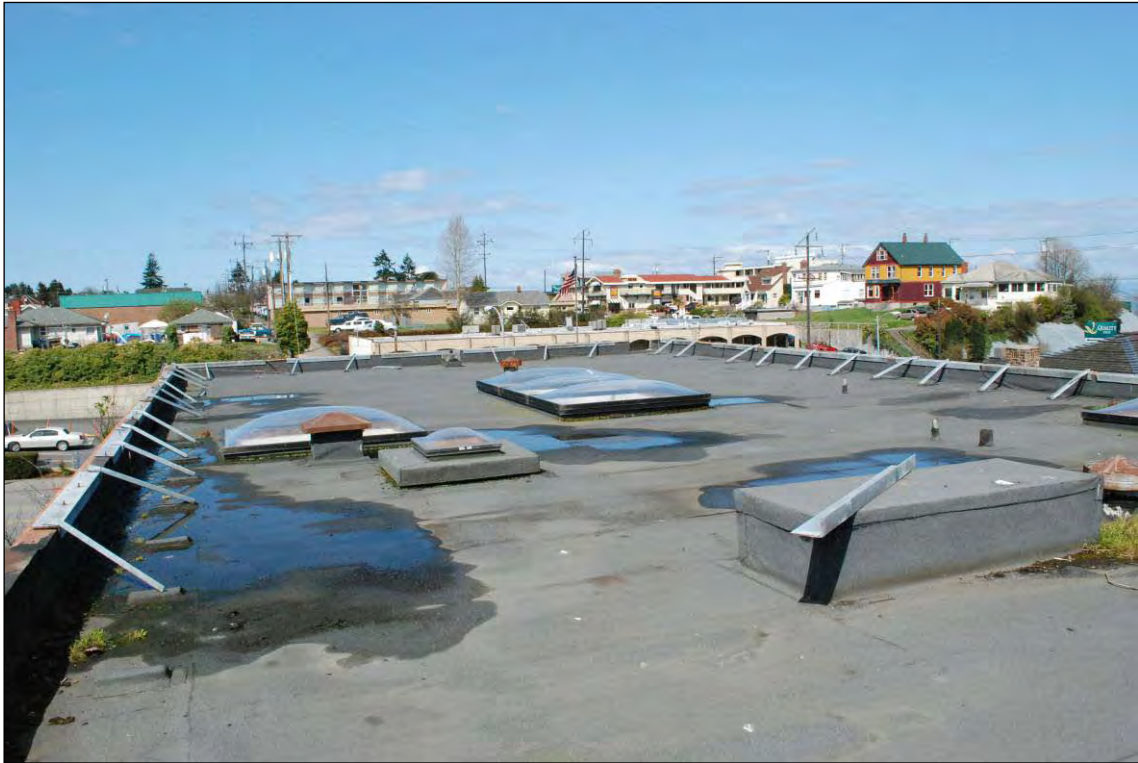
Figure 16 Above: Overall view roof looking west (April 2011)
