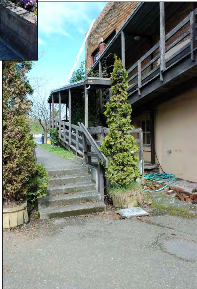
Figure 9 Below: View of freestanding wood access ramp, on the south side of the building looking north (April 2011)
