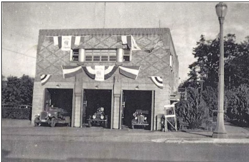
View of the Fire House with its doors opened.
