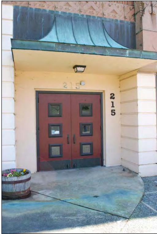
Figure 6 Above: View of main entry, west facade (April 2011)
