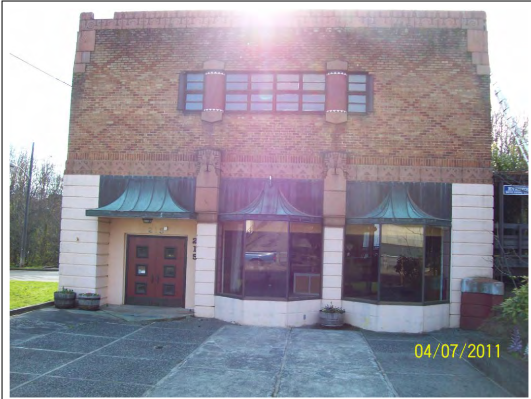
1. Main entrance to former firehouse. Several exterior paints were sampled to be tested as suspect LBPs.
