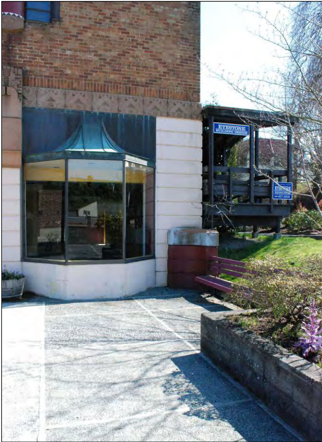
Figure 8 Left: Detail view of bay window, west façade, and freestanding wood access ramp (April 2011)
