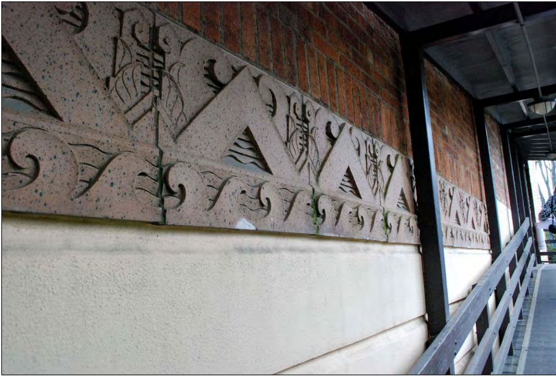
Figure 12 Above: Detail view of decorative terra cotta banding (April 2011)
