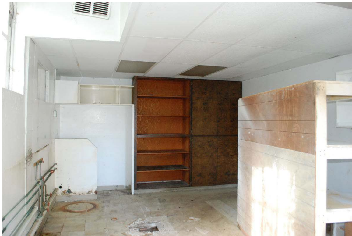
Figure 29 Below: Overall view of storage room at northeast corner of ground floor, looking south (April 2011)
