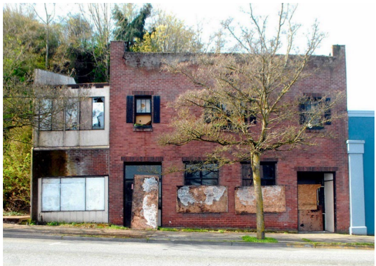
Figure 9. Razed Abandoned Building in the 200 Block of East Front Street
