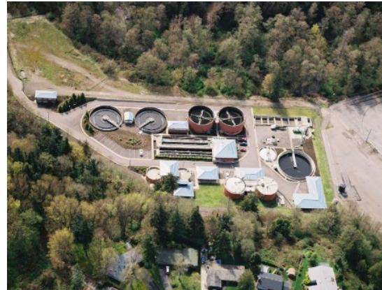
Port Angeles Wastewater Treatment Plant
