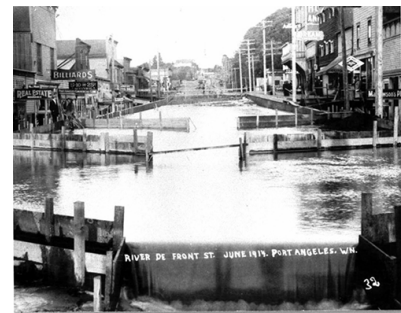
Downtown Port Angeles was dramatically transformed in 1914 when street-level grades were raised 12 feet or more following a massive sluice operation - effectively a man-made mud slide using a nearby hillside for source material.
