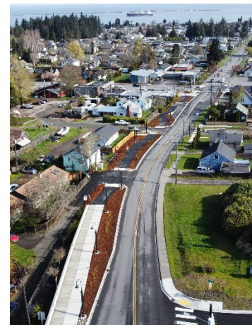
Race Street improvements
