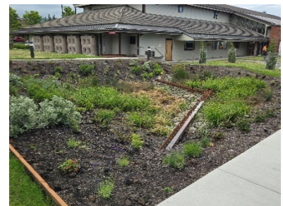
City Hall Bioretention pond
