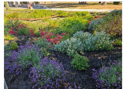
Bioretention pond (PWKS Engineering)
