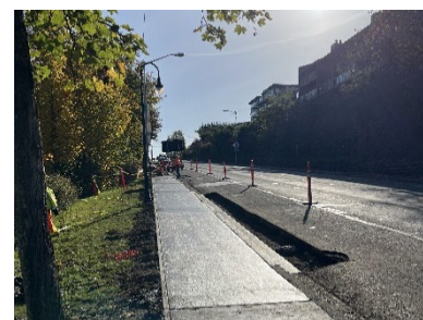
Downtown tree and sidewalk replacement (PKWS Engineering)
