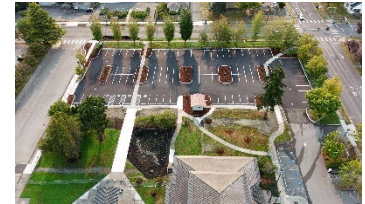
City Hall parking lot (PWKS Engineering)
