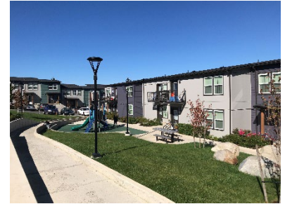
Multifamily housing in Port Angeles
