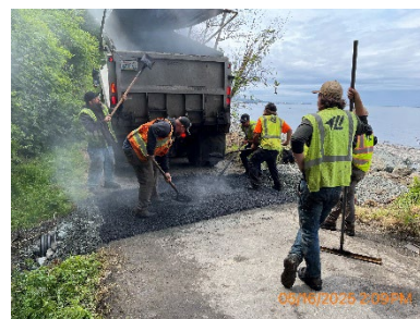
Olympic Discovery Trail upgrades (PWKS Engineering)
