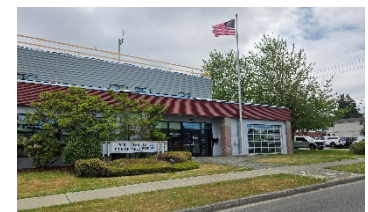
Port Angeles Fire Department
