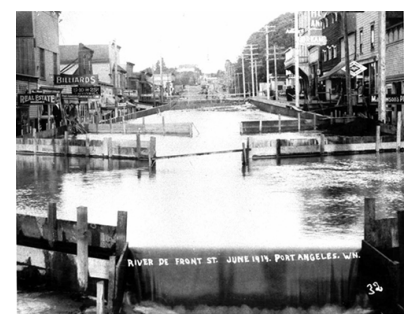
Downtown Port Angeles was dramatically transformed in 1914 when street-level grades were raised 12 feet or more following a massive sluice operation; this was effectively a manmade mud slide using a nearby hillside for source material.
