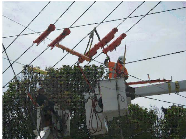
A little substation repair.
