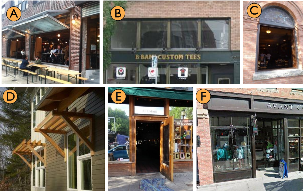
Examples of decorative or specially designed windows and entries. A = openable storefront window. B = transom windows. C = openable window with decorative details. D = decorative window shades. E = decorative door. F = recessed entry.
