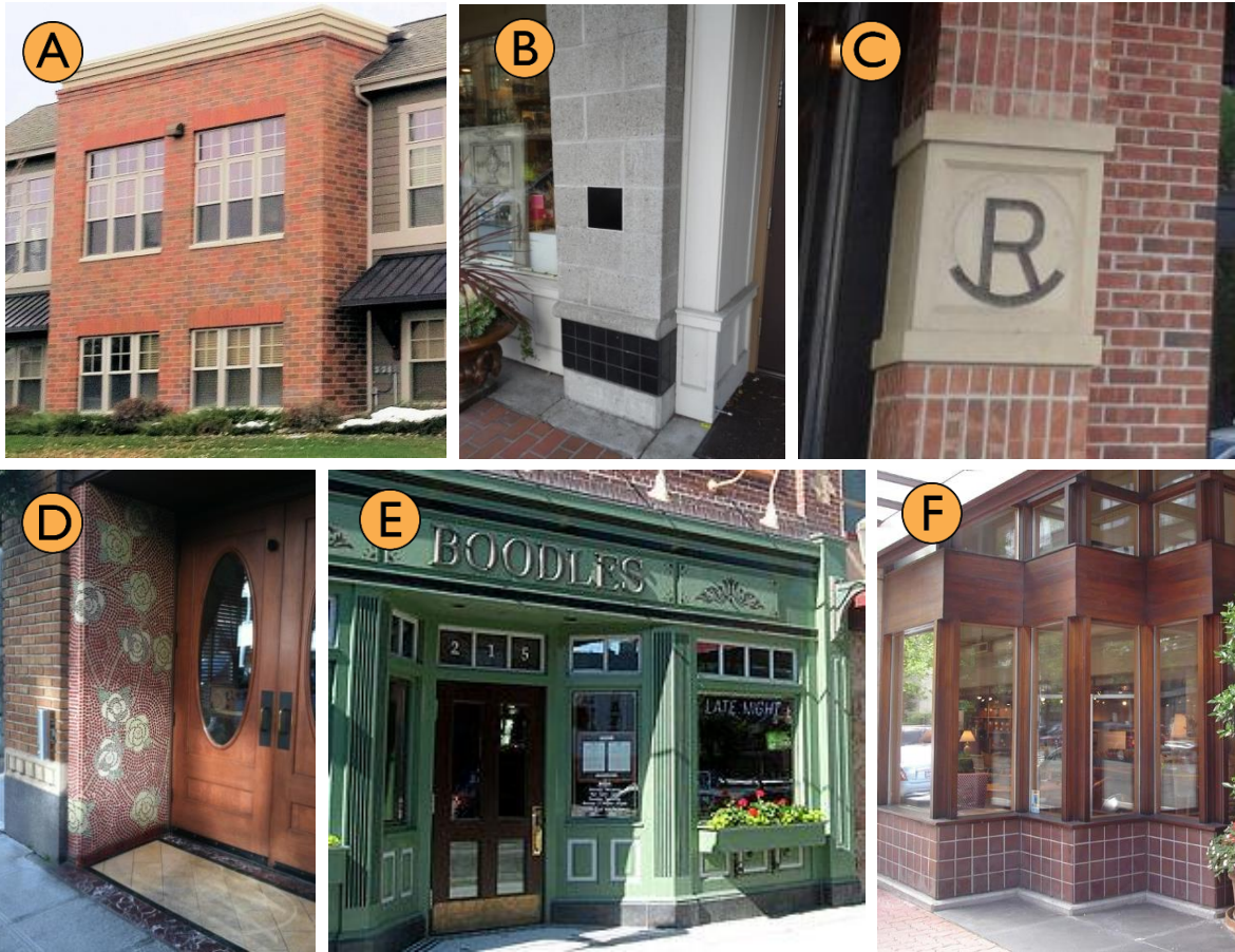
Examples of decorative surface materials. A = decorative brick/design. B = decorative tile-work and column pattern. C = decorative medallion. D = decorative mosaic tile work. E = decorative bulkhead. F = decorative materials and design.
