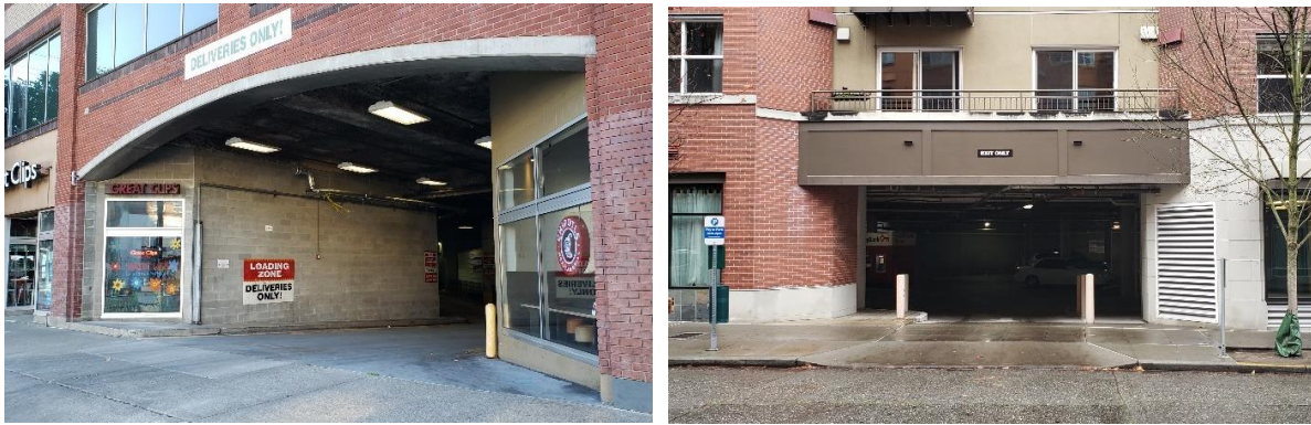
Left: This commercial/loading entry has cropped corners that are also utilized for store windows. Right: This residential garage has a setback and cropped corners on both sides that are also integrated into the design of the building façade above.
