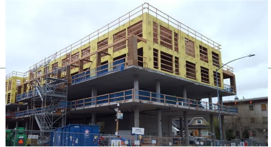
An example of wood-over-concrete construction that is common across the Pacific Northwest
