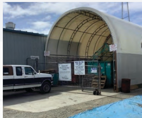
Centralized oil collection location. Putting all the oil collection and management devices in one location lessens the impact from oil sitewise and means that there is only one place to worry about when it comes to oil management.
