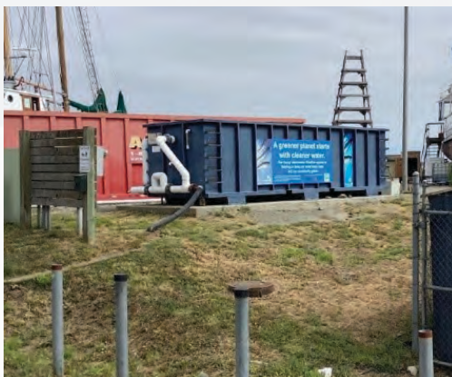
Centralized oil collection location. Putting all the oil collection and management devices in one location lessens the impact from oil sitewise and means that there is only one place to worry about when it comes to oil management.
