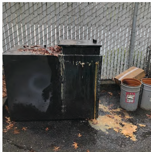
Before: Same photo from a different angle. You can see the clear signs of spillage on the container itself and the ground next to the container.
