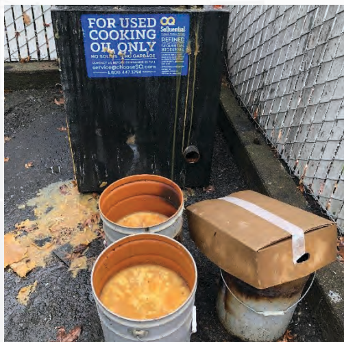
Before: Fats, oils, and greases (F.O.G) being stored in open-top 5-gallon buckets. This type of storage increases the likelihood of spills to the environment. In this photo, you can see spilled F.O.G. next to the containers.
