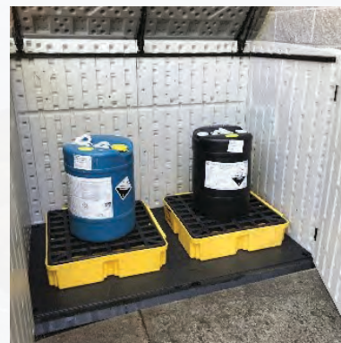
After: The new covered storage with secondary containment for chemical management.
